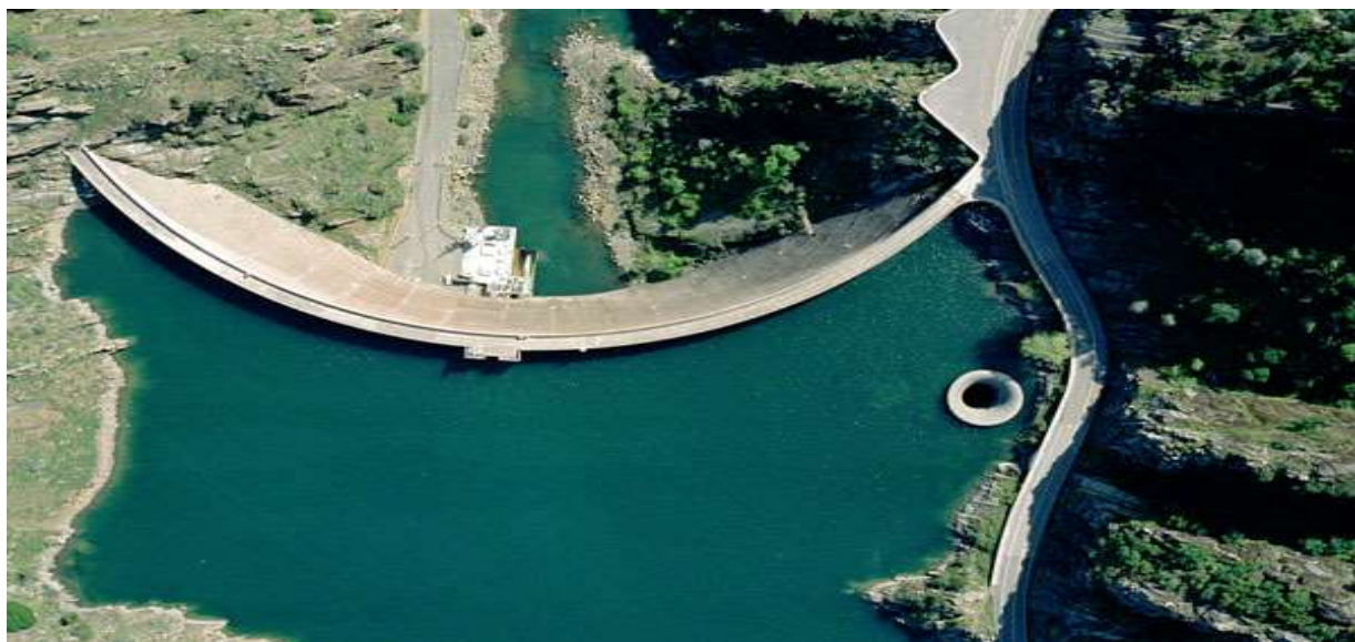
Overhead view of Monticello Dam and Powerhouse
