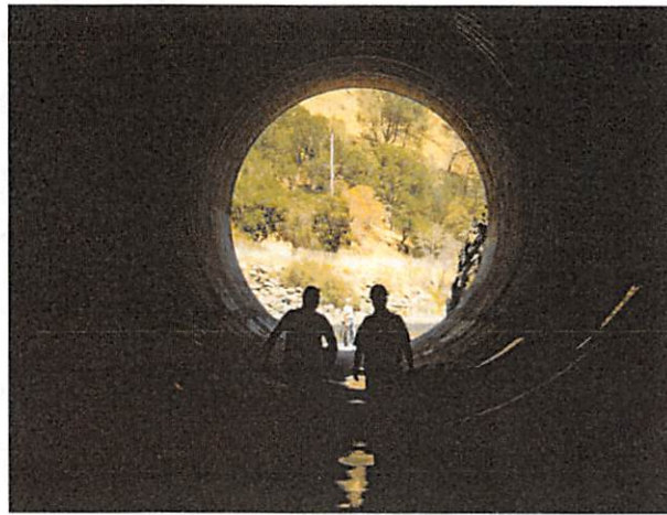
Glory Hole Spillway Outlet
