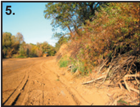
5. Out-of-place channel after fill and initial grading.
