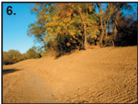
6. The out-of-place channel after fill and slope applied toward Putah Creek Road. Seeding was completed after this image was recorded.
