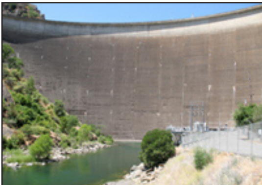
Monticello Dam monitoring site.
