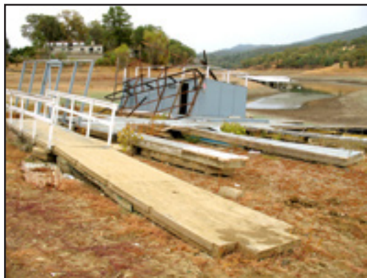
Abandoned Dock. Putah Creek Resort. Lake Berryessa. October 2008.
