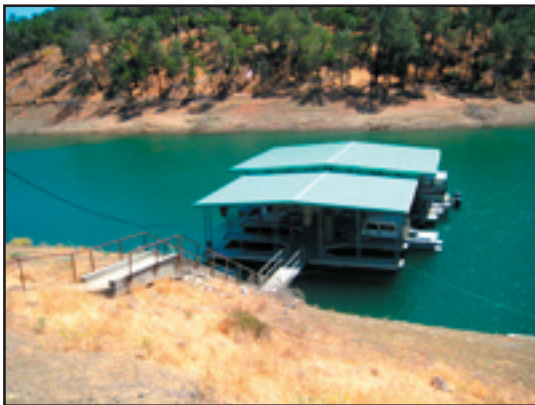
Lake Berryessa. Headquarters' Cove boat dock.
