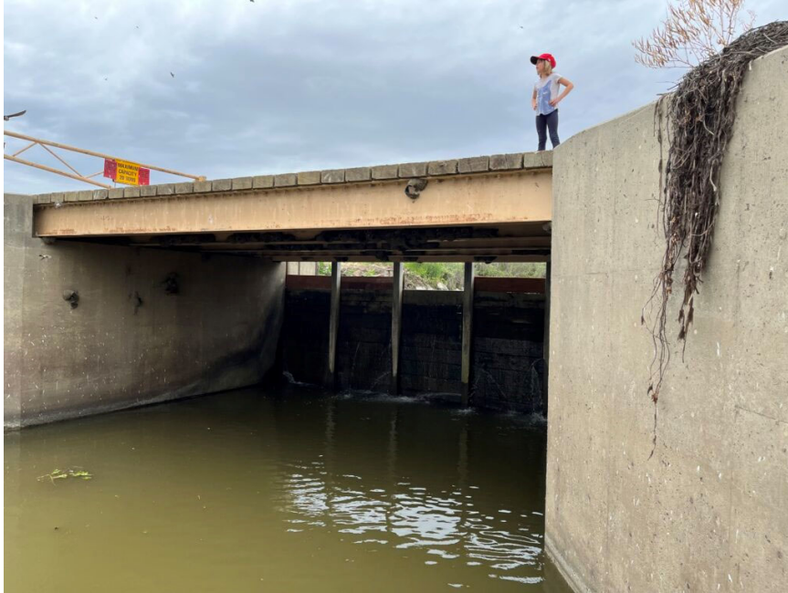
Check dam with manual
