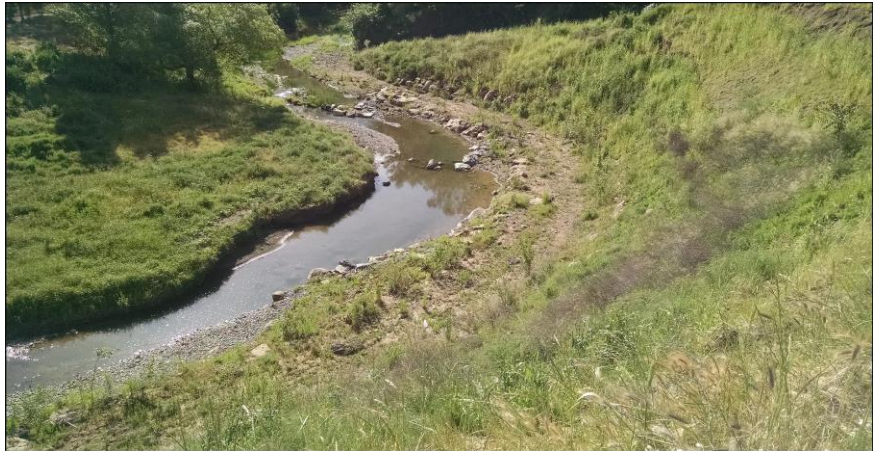
Figure 2: Same location as Figure 1. Photo taken one year after project completion and implementation of rock vanes, installation of a bench at floodplain elevation which reduced the slope of the bank facilitating the growth of vegetation and minimizing erosion.
