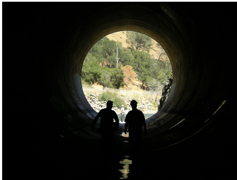
Glory Hole Spillway Outlet
