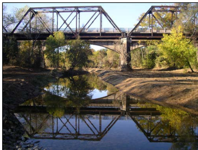
Winters Putah Creek Park Restoration Project Photo credit: Thomas Pate
