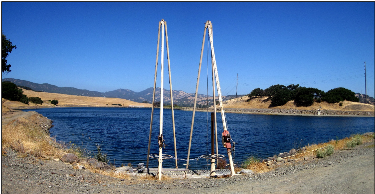
Putah South Canal Terminal Reservoir, Solano Project
