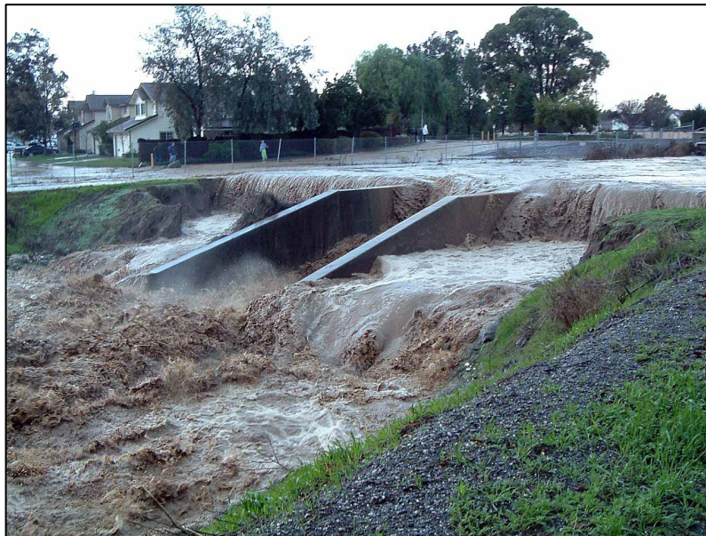
Ulatis Flood Control Channel at Nut Tree Road, Vacaville (Dec 2005)
