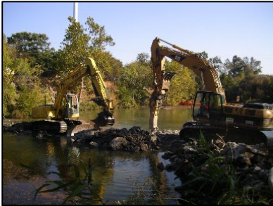
Putah Creek dam removal Creek restoration site
