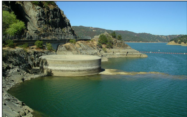
“Glory Hole” Spillway at Lake Berryessa (2008) – 28 ft. diameter
