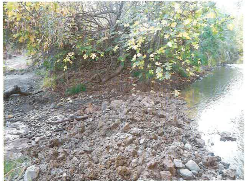
Channel Plug at NAWCA 3
